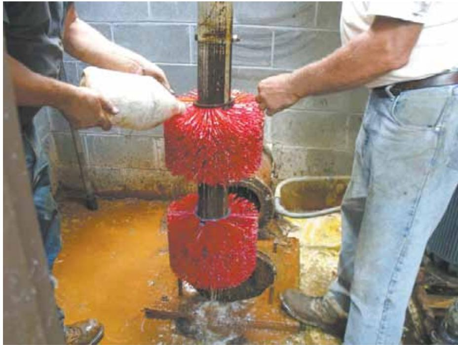
The most basic mechanical method of rehabilitation is simply running a brush down the hole and scrubbing the inside of the casing wall. *Source: Cotey Chemical photos.*
